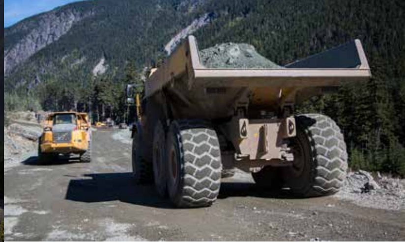
Clare Forest Service Road construction east of Mount Nimbus.
