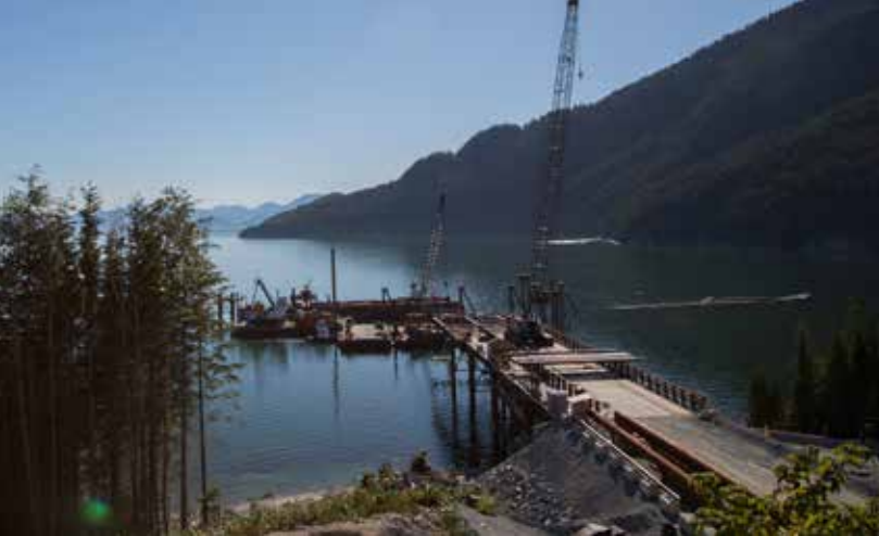
Marine trestle at the Bish Cove Kitimat LNG plant site.
